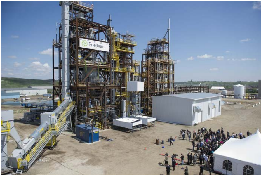
Figure 3-1 Preliminary Photo: Enerkem Facility in Edmonton
