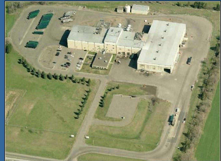
Resource Processing Plant (ER-RPP)
