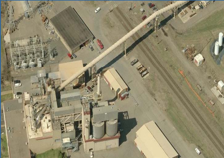
Energy Recovery Station (ER-ERS)
